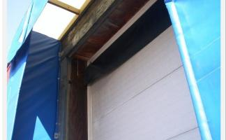
Rigid head frame is peaked to prevent snow and water build-up and covered with white vinyl to allow light in.
